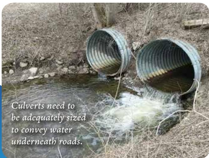
*Culverts need to be adequately sized to convey water underneath roads.*
