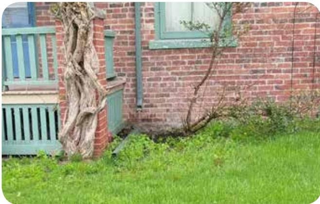
*Homes can be at elevated risk of flooding from downspouts discharging at the foundation, something which can be easily fixed.*
