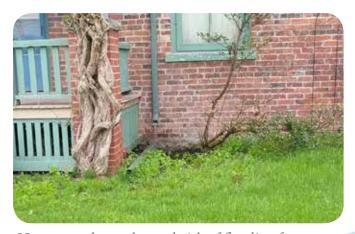
Homes can be at elevated risk of flooding from downspouts discharging at the foundation, something which can be easily fixed.
